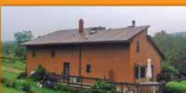
Asphalt Shingle and Metal Roofing
